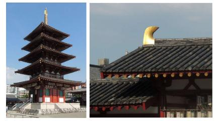
Figure 15. Lightning rod on pagoda (left) and roof horns on temple (right)
