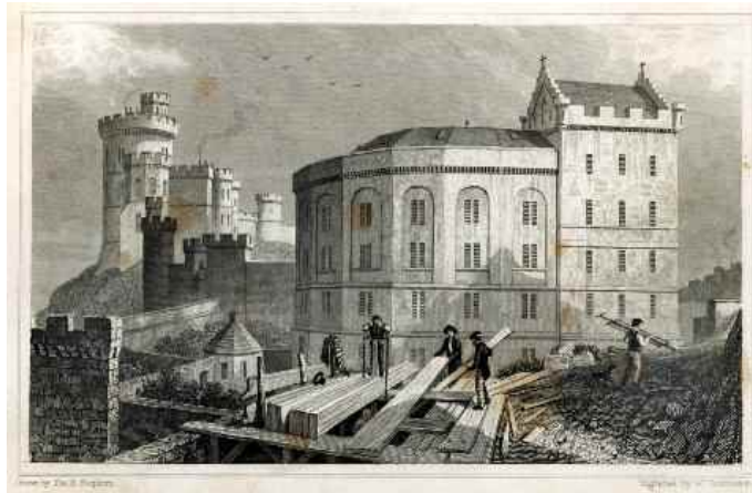
Figure 2.1.5 Edinburgh Bridewell During Construction 94
