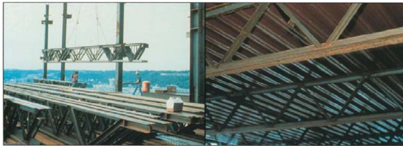
Figure 3.3.3 Vulcraft Open-Web Joist 309
