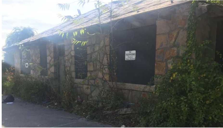
Figure 2.3: Exterior view of the existing structure (East Wall)
