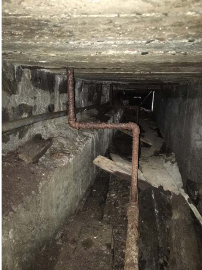
Figure 2.5: Crawl space next to foundation of existing building
