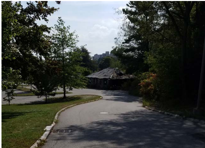
Figure 2.1: Entrance to the site with the existing building
