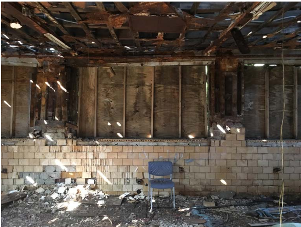
Figure 2.4: Interior of the existing building
