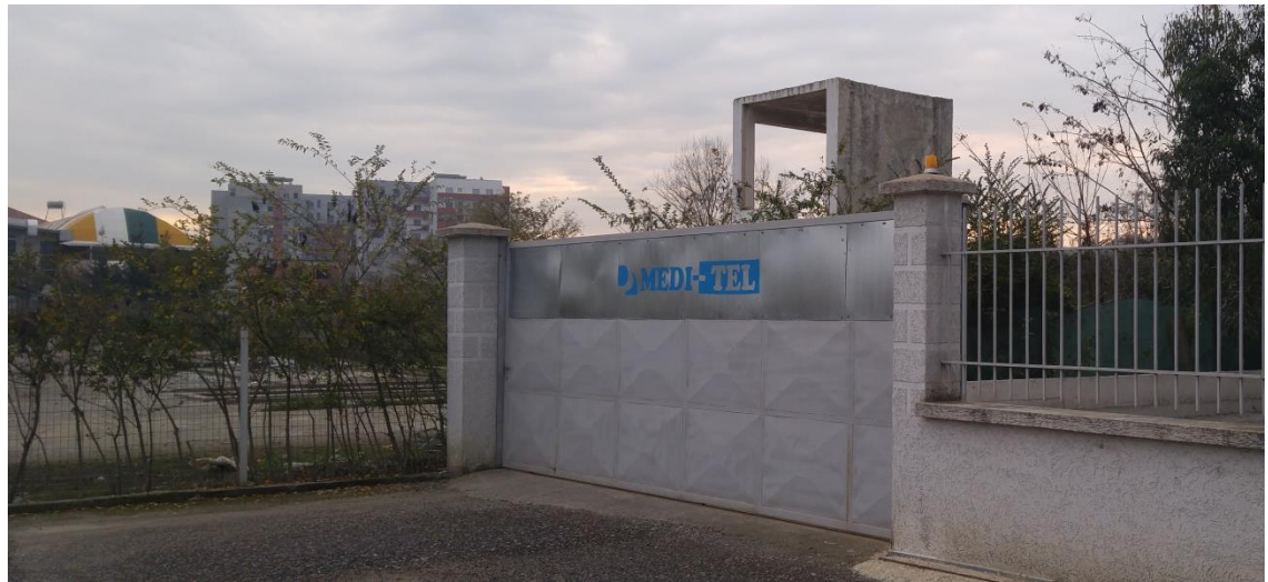
Figure 11: Medi-Tel Treatment Facility
