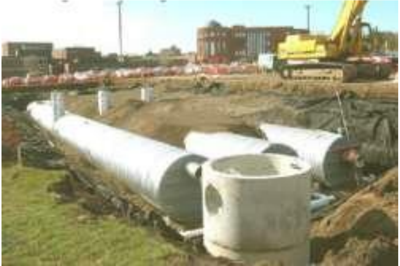
Figure 1: Subsurface Detention System (Underground Storage)
