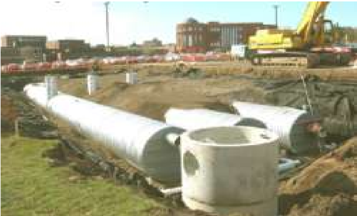
Figure 5: Subsurface Detention System
