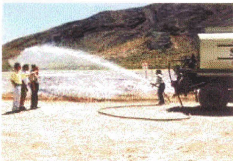
Figure 1(a) – Applying a Dust Suppressant ( http://www.lasvegas.com/realestate/REAug-09-Sun-1998/Front/7929616.html ) Tank truck with hose for manual spray.
