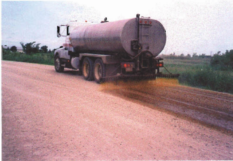
Figure 1(b) – Applying a dust suppressant ( http://www.usroads.com/journals/rmej/9806/rm980604.htm ) Tank truck applying suppressant with rear distribution bar
