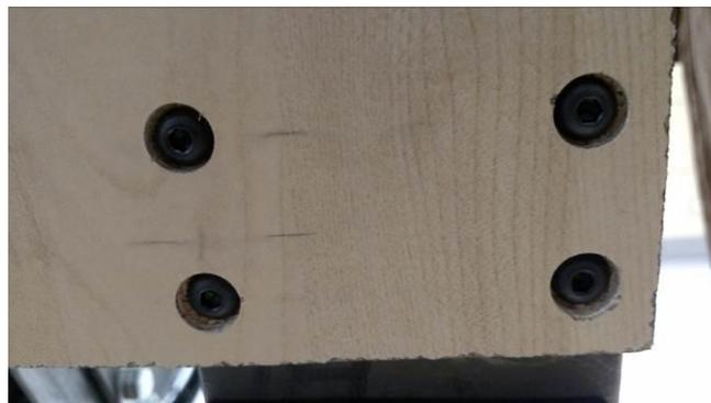
**Figure 42: Sample of counter-bore Holes constructed within the front board.**
