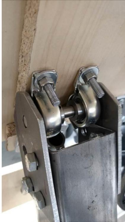
**Figure 41: Center Beam Pivoting Connection.**
