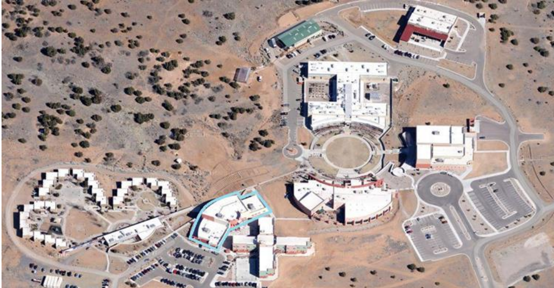
Figure 14: Aerial view of the IAIA campus. The CLE building is outlined in blue.
