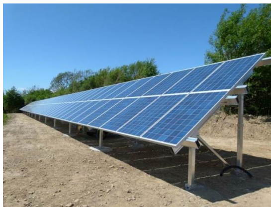
Figure 10: An example of a ground-mounted solar array 76
