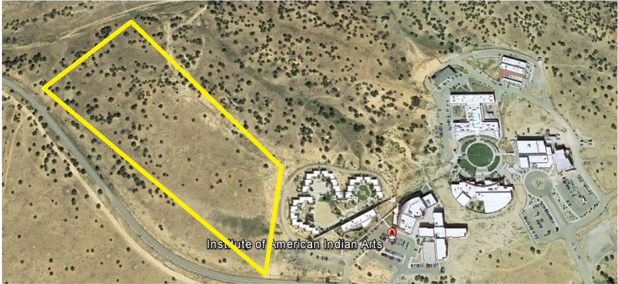
Figure 23: Outlined in yellow are possible areas that ground-mounted solar panels can be installed.
