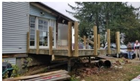
Figure 6: House under repair in Marlborough (Community Advocate, 2017).
