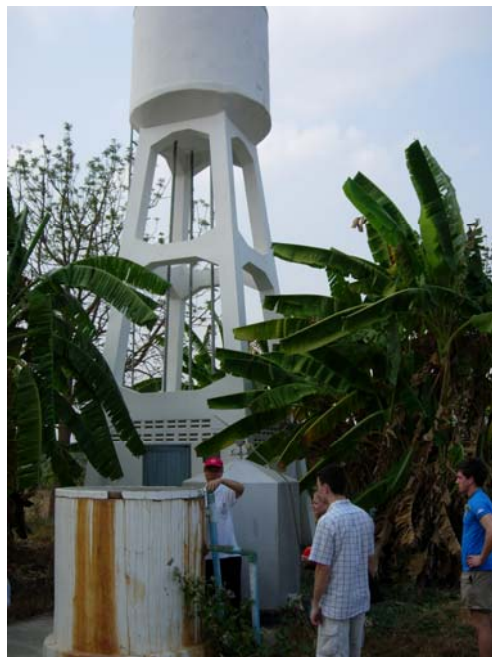
Photograph 2: Water tower irrigation system at New Life
