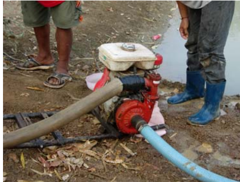
Photograph 16: Pumping reservoir water directly into the main line
