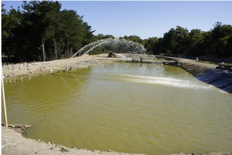
Figure 12. Leachate aeration at Grantville facility.
