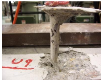
Figure 39: Uncleaned HIT RE-500 Pulled Out Anchor
