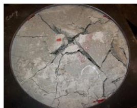
Figure 27: Concrete Failure, HIT RE 500 Cleaned
