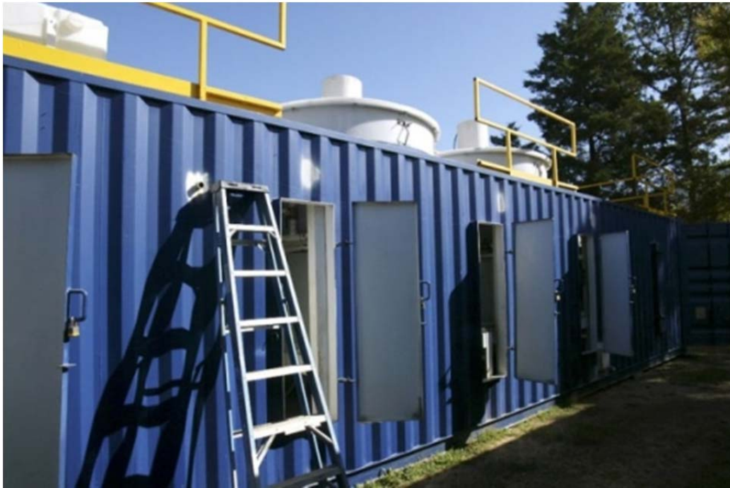
Figure 23: The Waste Treatment Plant (Clark).
