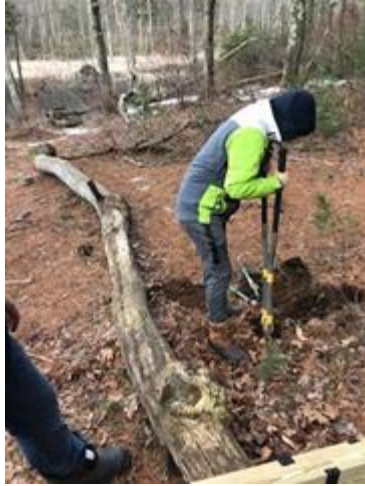
Figure 30. Digging of Post Holes
