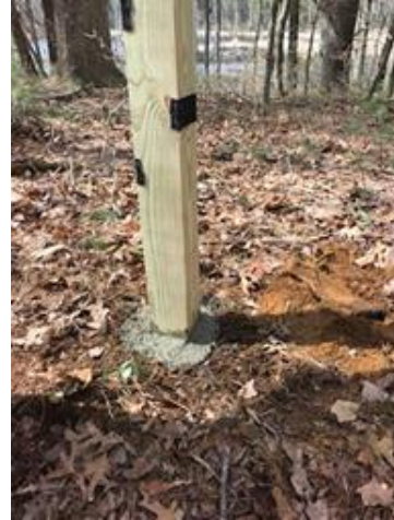
Figure 31. Cemented Post
