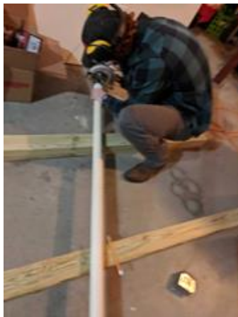
Figure 26. Cutting of PVC Pipes
