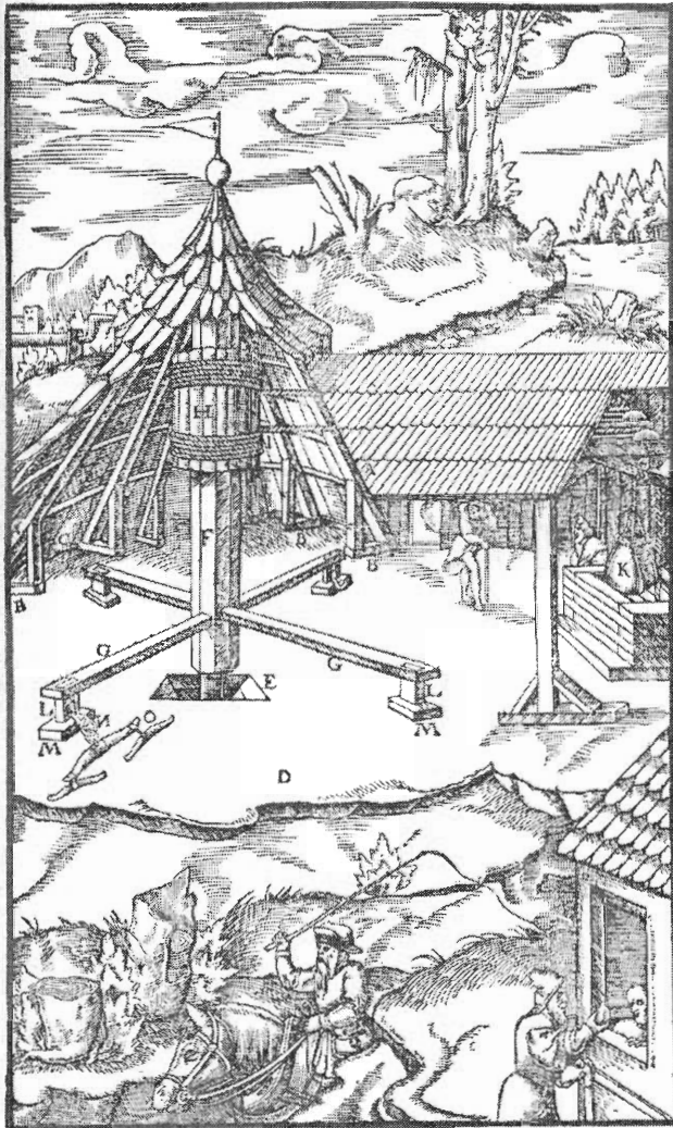
A—UPRIGHT BEAMS. B—SILUS LAID FLAT UPON THE GROUND. C—POSTS. D—AREA. E—SILL SET AT THE BOTTOM OF THE HOLE. F—AXLE. G—DOUBLE CROSS-BEAMS. H—DRUM. I—WINDING-ROPE. K—BUCKET. L—SMALL PIECES OF WOOD HANGING FROM DOUBLE CROSS-BEAMS. M—SHORT WOODEN BLOCK. N—CHAIN. O—POLE BAR. P—GRAPPLING ROOK. (Some members mentioned in the text are not shown).
