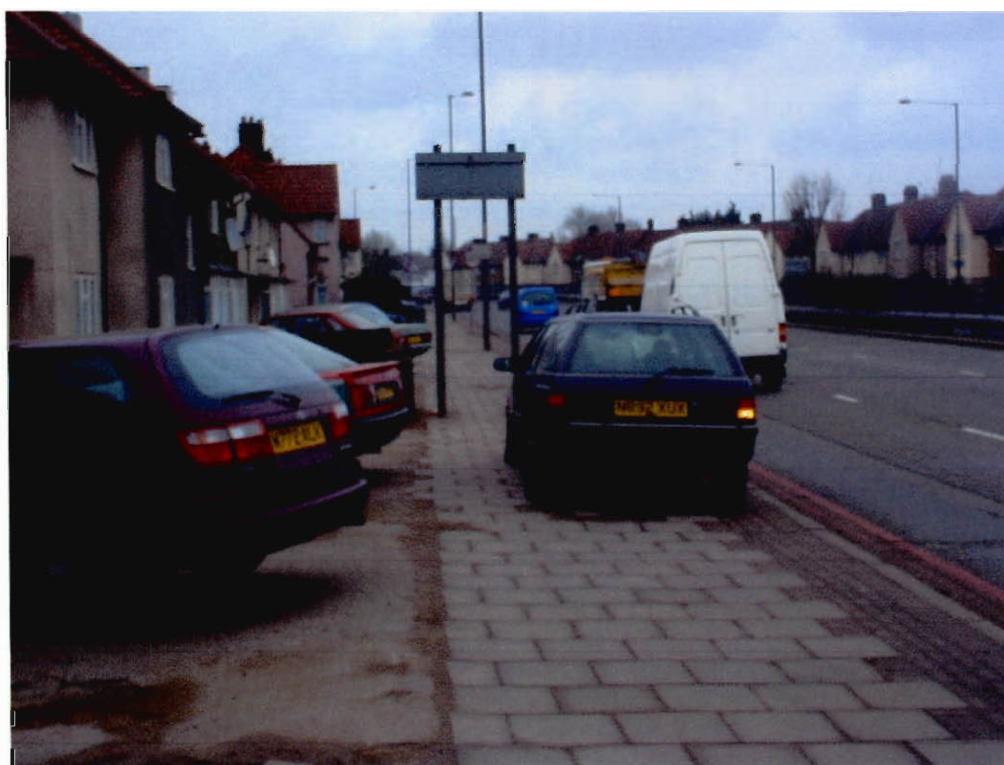
Figure 2.12: Narrow sidewalk along NCR
