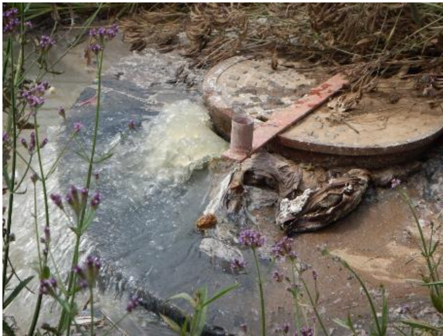
Figure 17 - Uplifted Manhole
