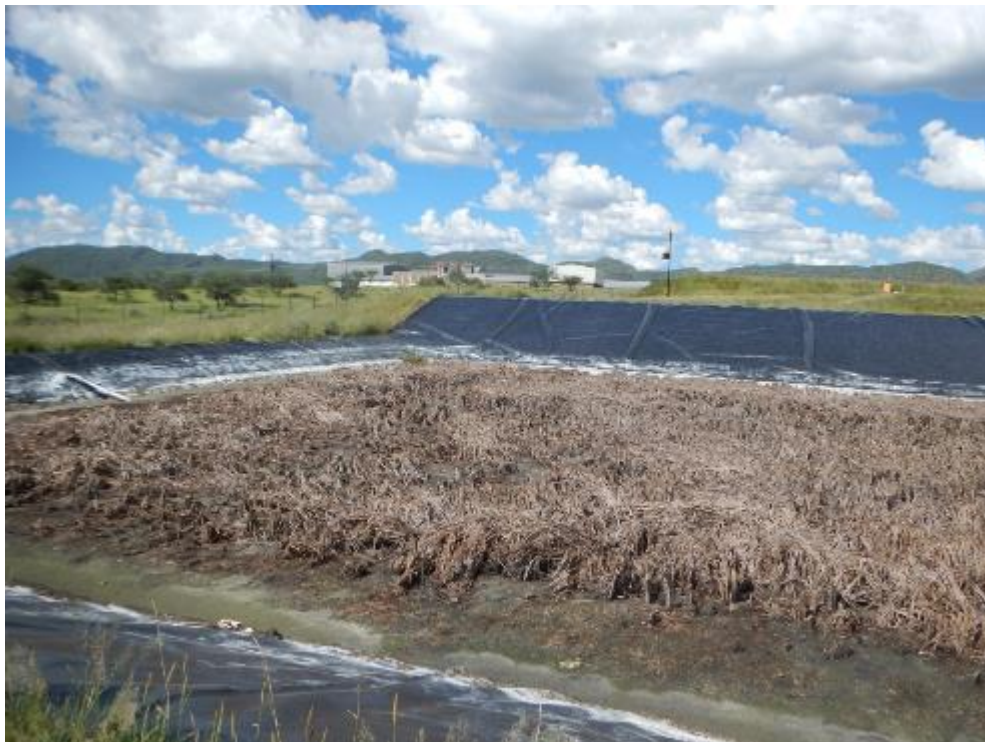
Figure 19 - Ineffective Water Treatment Stage - Namib Poultry
