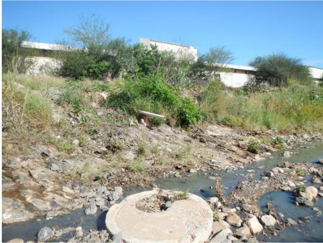
Figure 20 – Illegal Waste Disposal
