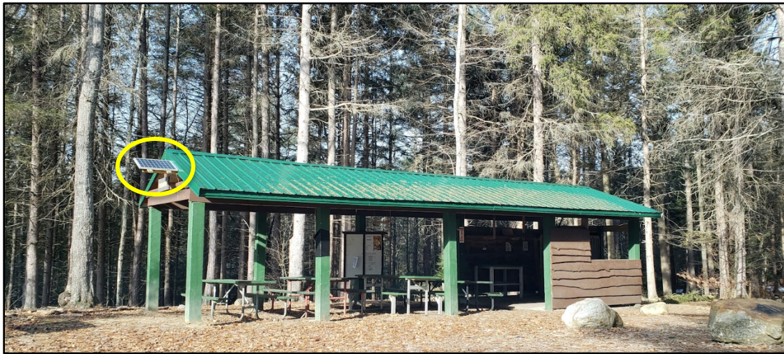
Figure 1: Camp Hard Shelter with Solar Installment (Yellow)
