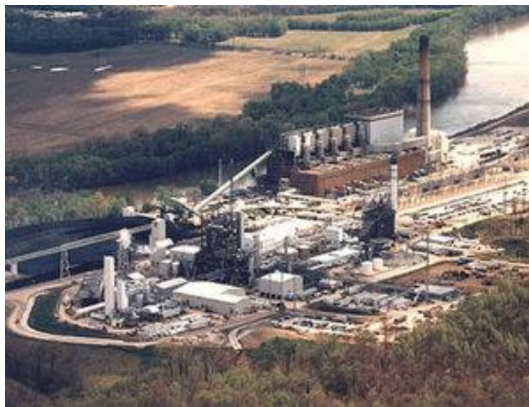
Figure 10: Wabash Power Station 19
