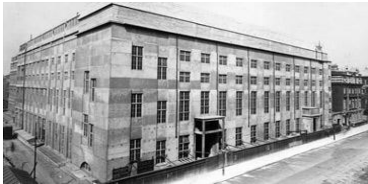
Figure 1: The East Block of the London Science museum during construction in 1919 (Science Museum, "Construction," n.d.)
