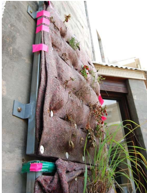
Figure 6: An example of a modular fabric living wall. " mobbs' vertical garden " by nicolas.boullosa is licensed under CC BY 2.0 .
