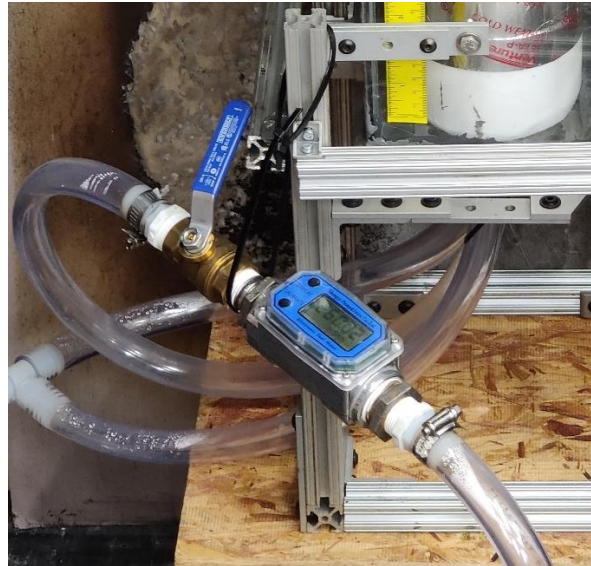
Figure A1. 4: The pipelines and control valve in the turbulence generation system.
