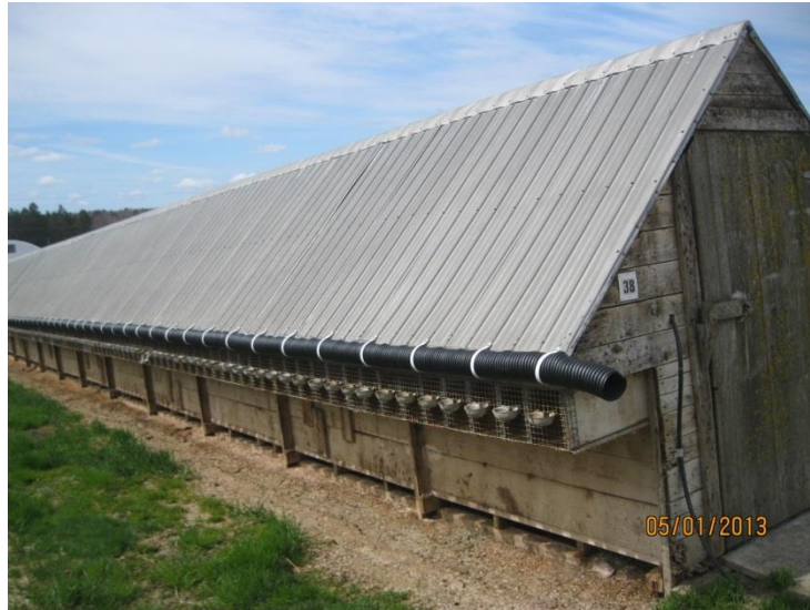
Figure 1: Traditional mink Farming Structure. Notice the cages hanging out over the ground. Photo taken by Stantec.
