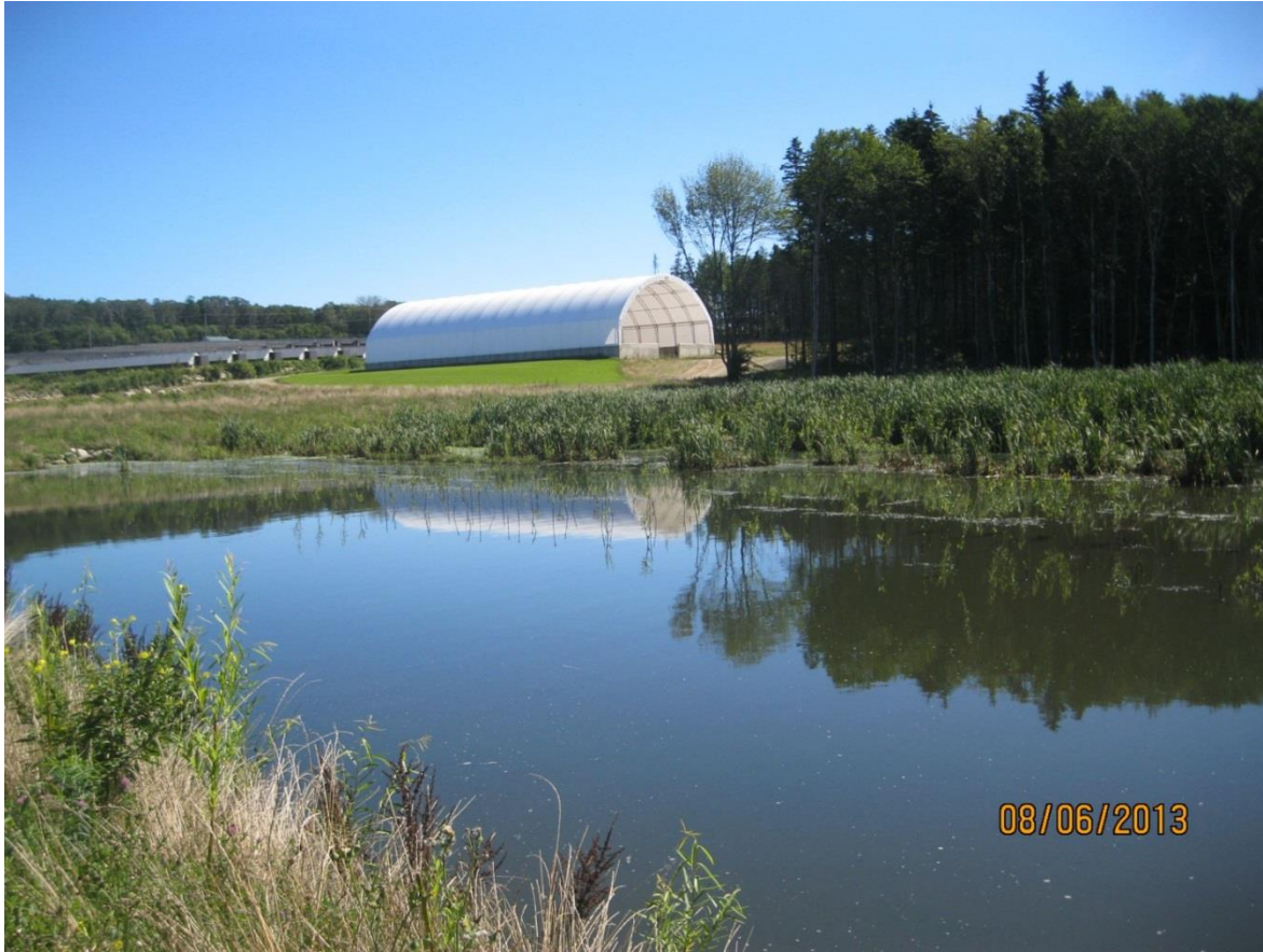
Figure 18: Manure Storage Building. Photo Taken by Stantec
