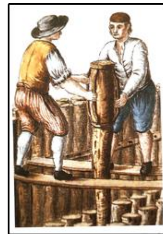
Figure 2. Venetians Building Wooden Foundations 6
