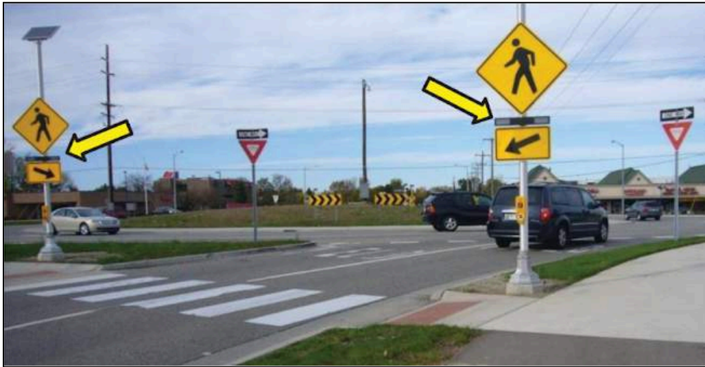
Figure 29. Example of RRFBs at crosswalks in a roundabout in Oakland County, Michigan (Schroeder et al., 2017).
