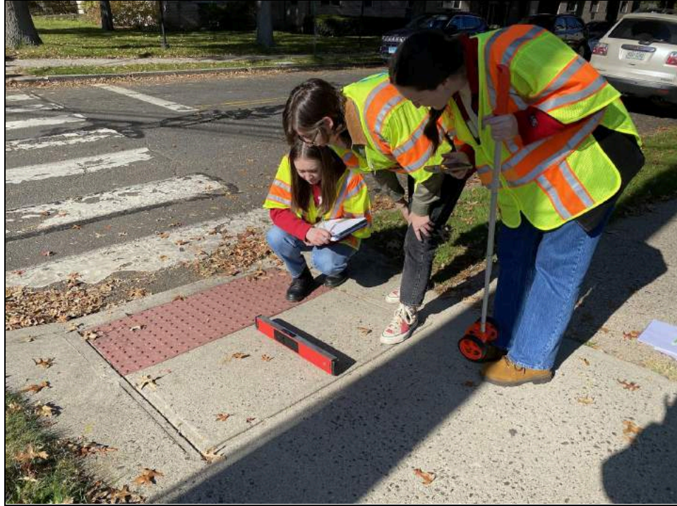
Figure 3. The team conducting a curb ramp inspection (#11 curb ramp) on Cartright St.
