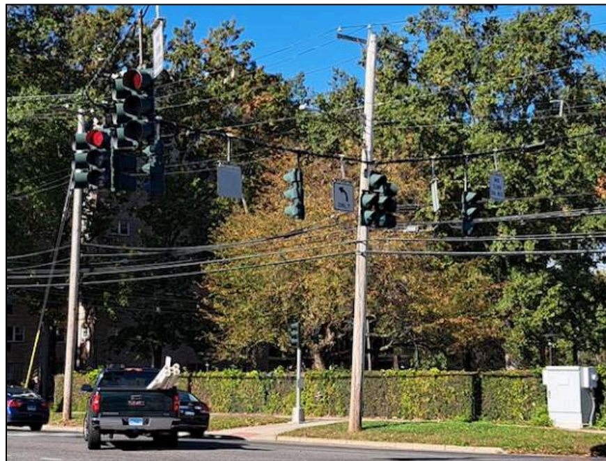
Figure 13. Poor sightlines to traffic signals for pedestrians.
