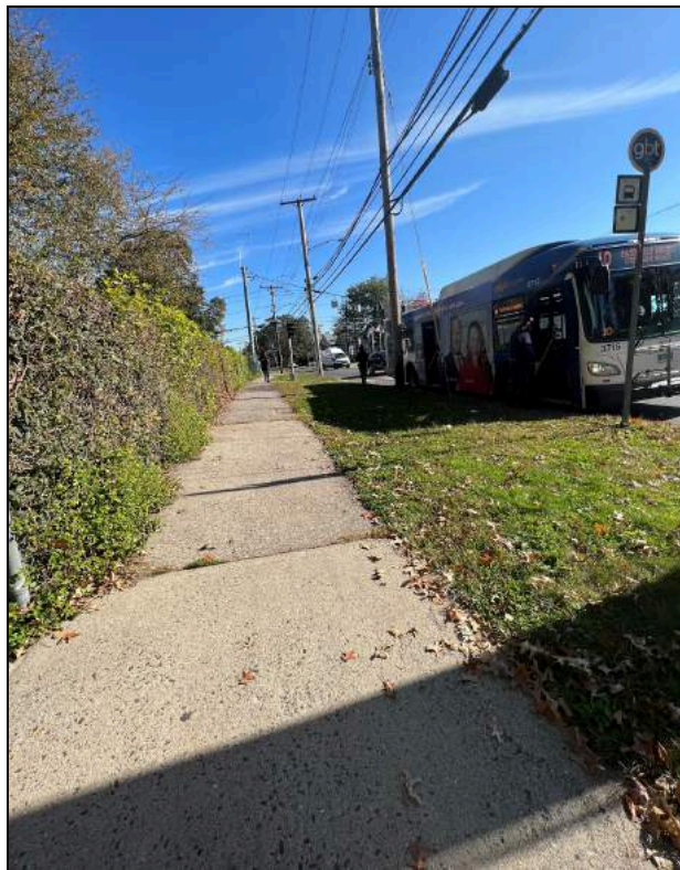
Figure 19. Inaccessible Bus Stop Access Route.
