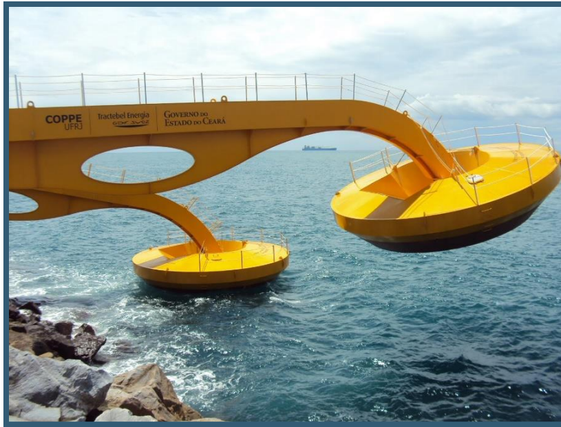
Figure 5: Wave energy harvester from SDE ltd. [26]
