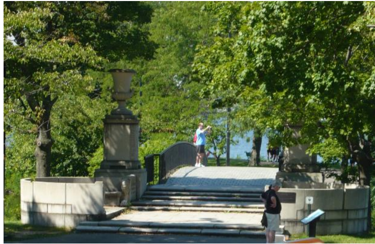
Figure 16 - Bridge at the Charles River Esplanade that could have a technology counter to be used as a focal point.
