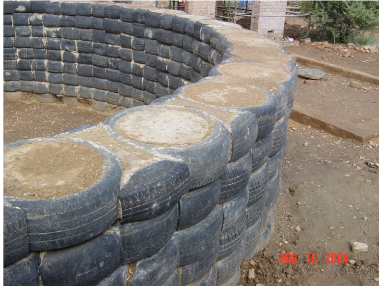
Figure 8: Tyres used as a building material for walls at the HRDC
