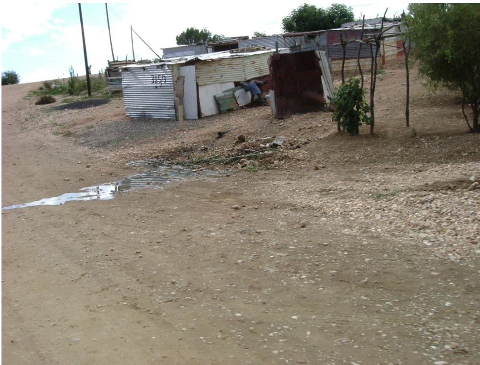
Figure 3: Improper drainage of makeshift structures conducive to grey water surface pools in the Northwest Settlements (16 March 2004)
