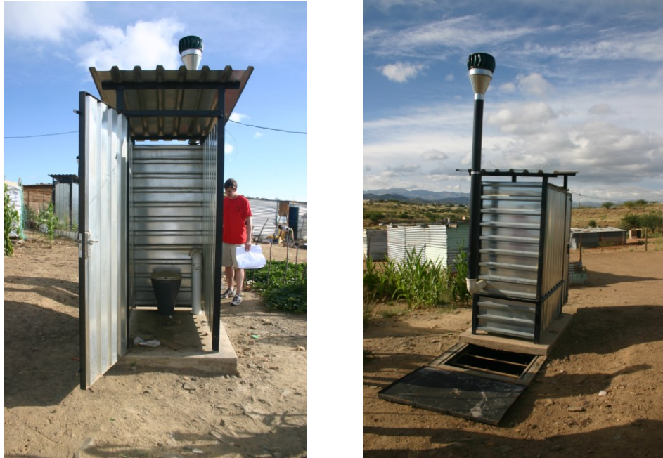
Figure 27: Inside and outside view of Cool Maintenance dry toilet facility with the sewage pit cover opened
