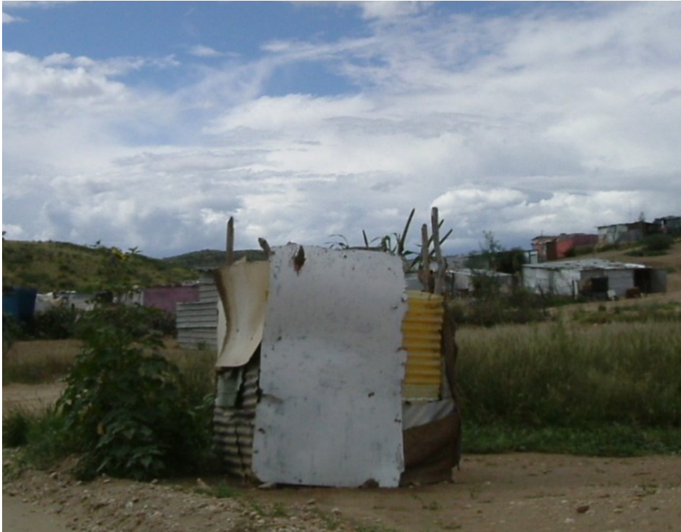
Figure 2: A typical makeshift shower structure used by the settlers of the Northwest Settlement (16 March 2004)
