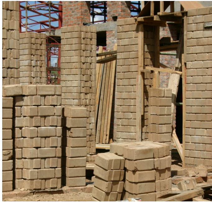
Figure 6: Interlocking bricks to be used for the walls of the Habitat Research and Development Centre
