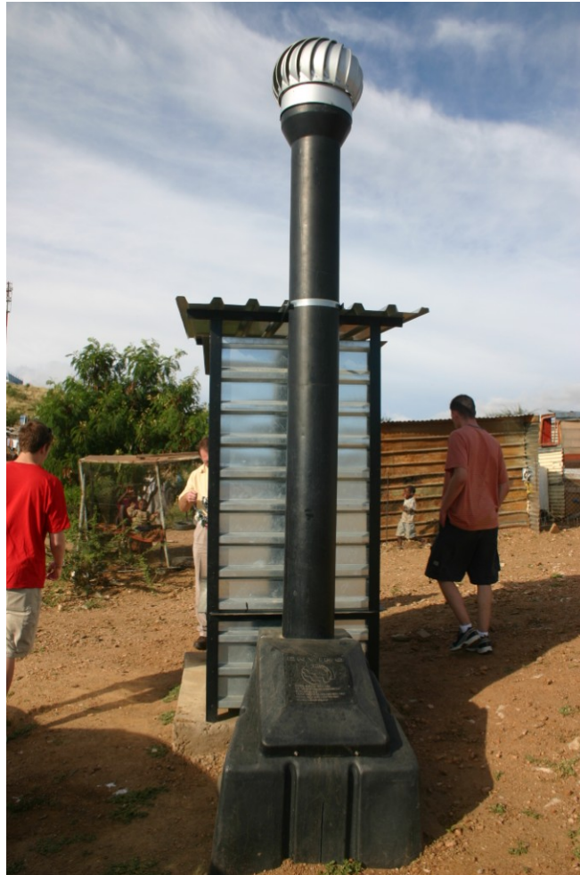
Figure 26: Corrugated iron toilet facility implementing the Enviro Loo design in Okahandja Park (31 March 2004)
