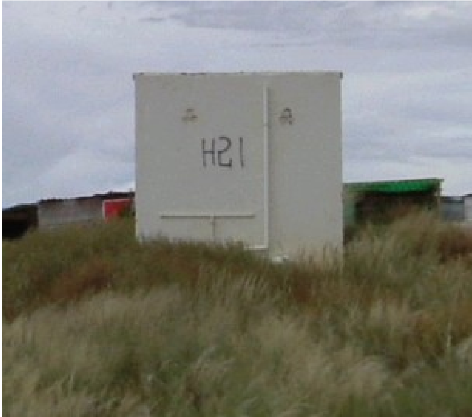
Figure 1: Toilet facility constructed in the Northwest Settlements (16 March 2004)
