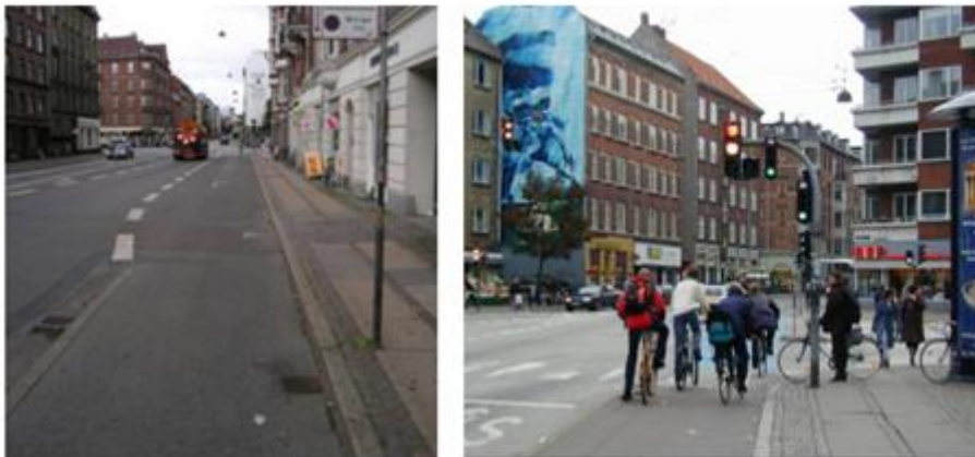
Figure 4: Photos of shortened bicycle track (left) and advanced bicycle track (right) (Jensen, 2008).
