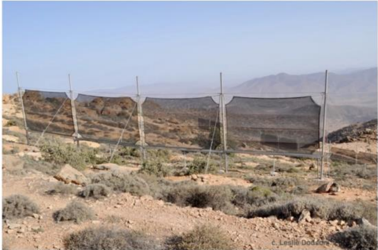
Figure 1. Fog water net set up in the Anti-Atlas Mountains of Morocco. Photo: Leslie Dodson (Dodson & Bargach 2015).
