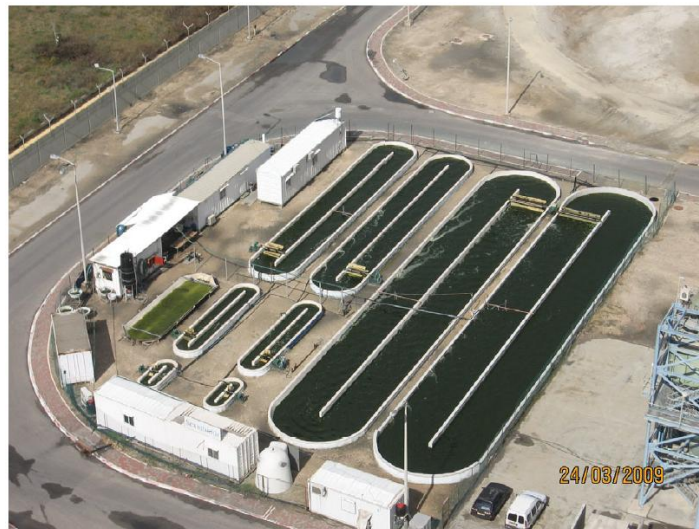
Figure 7: Example Open System Raceway Pond (Greenwell et al., 2010)
