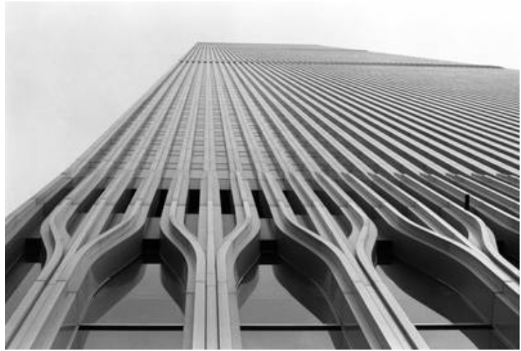
Figure 25: Structural Framed Envelope (Craven)
