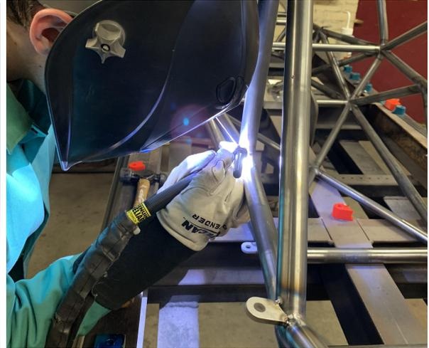
Figure 32: *Welding tabs onto frame.*
