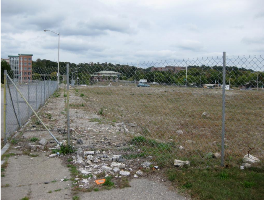
Figure 35: Pit at the 1 Concord Street site
