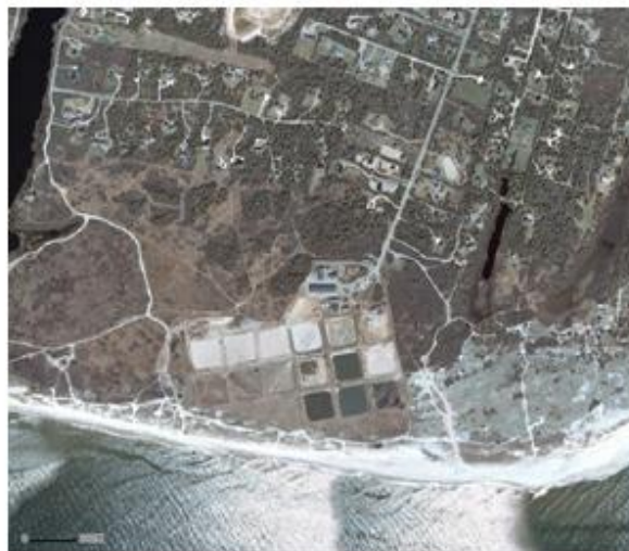
Waste Water Treatment Facility, Surfside
