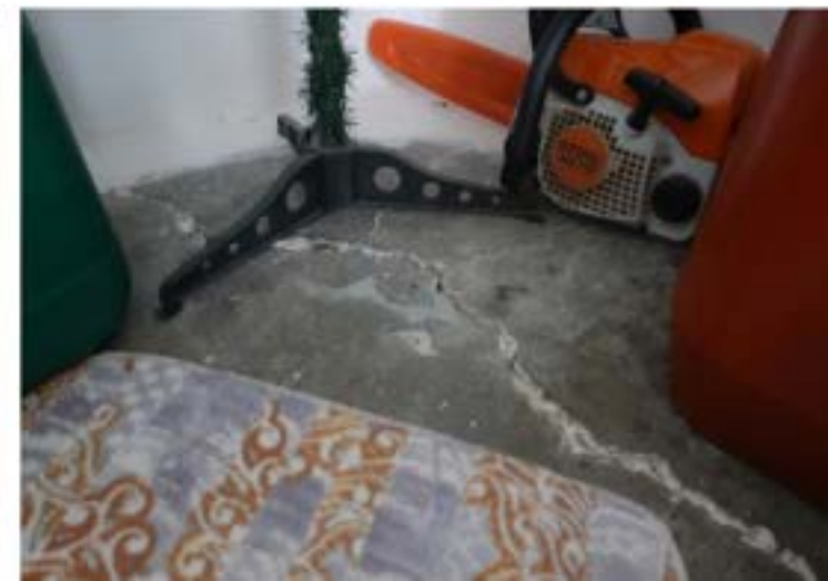
Figure 25 - Unfinished room in Sofie Senko's home after her roof collapsed in 2012-2017 tremors (left) Fiqerete Gremi's bedroom with large cracks in the walls and ceiling (middle) Crack in the concrete floor of Beruzë's livingroom (right) (own photos).
