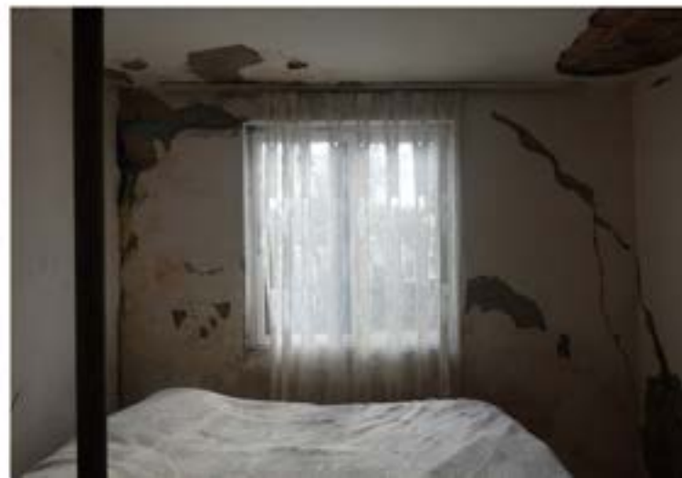
Figure 25 - Unfinished room in Sofie Senko's home after her roof collapsed in 2012-2017 tremors (left) Fiqerete Gremi's bedroom with large cracks in the walls and ceiling (middle) Crack in the concrete floor of Beruzë's livingroom (right) (own photos).
