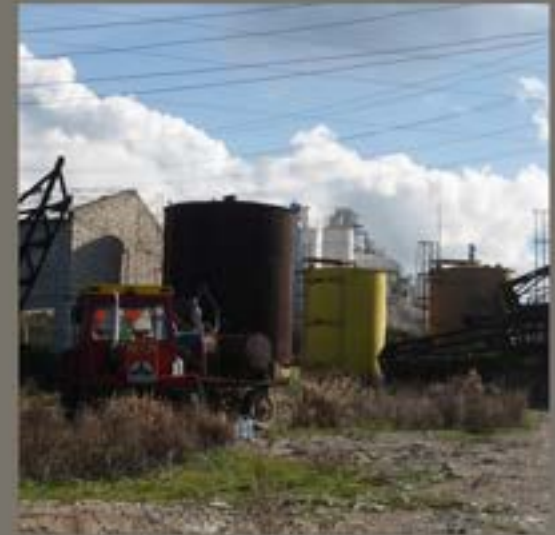
Processing tanks, truck, and discarded oil derricks (own photo)
