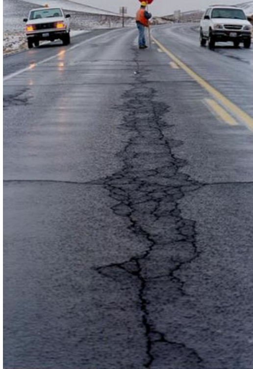
Figure 3: Fatigue cracking
