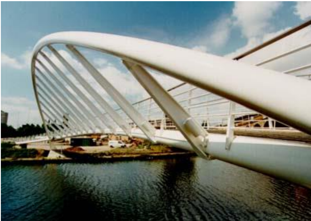
Figure 7: Merchants Bridge, Manchester, Great Britain
