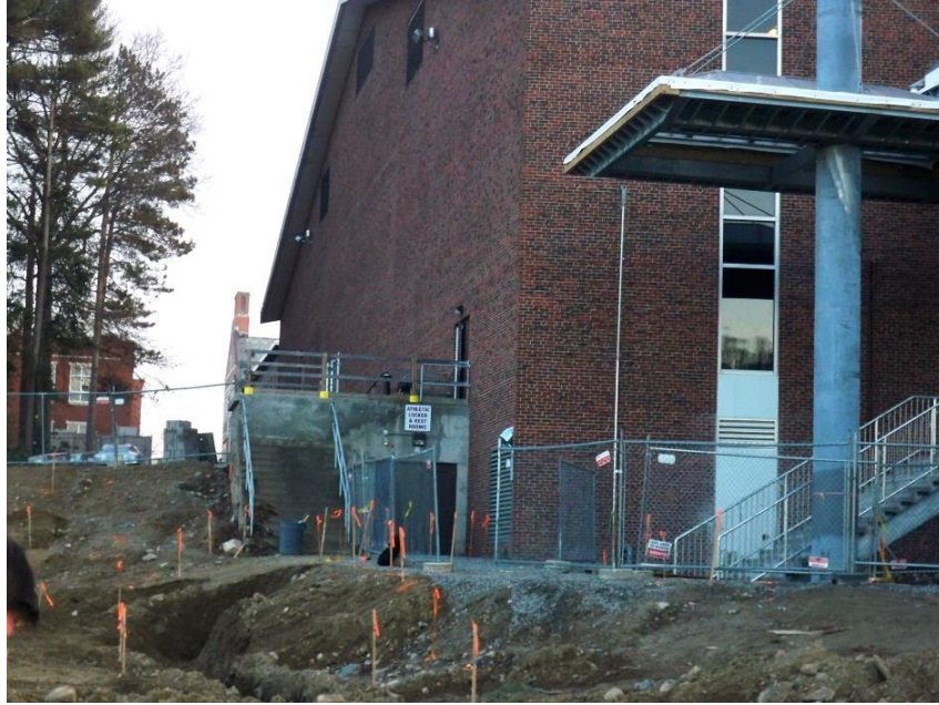
Figure 26: The Bridge Decking will meet with the Loading Docks behind Harrington
