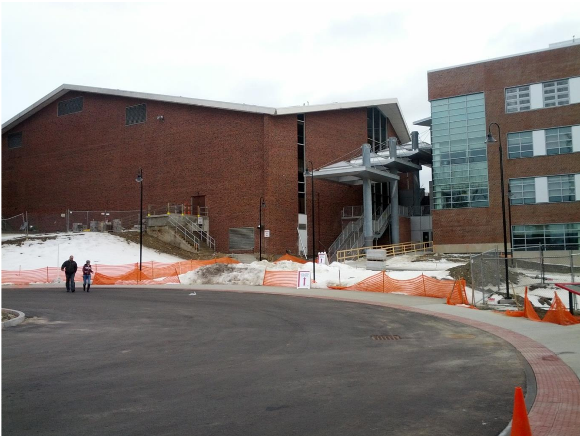
Figure 21: Looking Towards the Loading Dock
