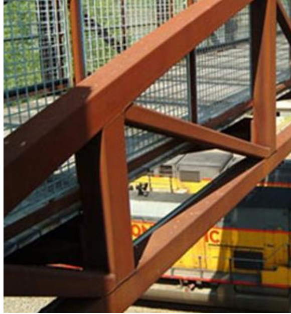
Figure 38: Typical Welded steel Connection
