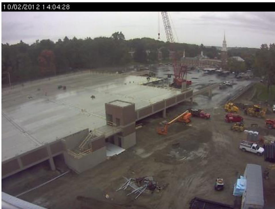
Figure 23: Garage in construction, showing area of interest for foundation
