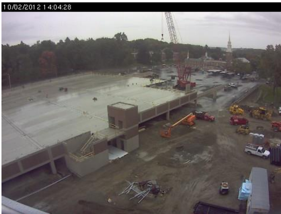
Figure 23: Garage in construction, showing area of interest for foundation
