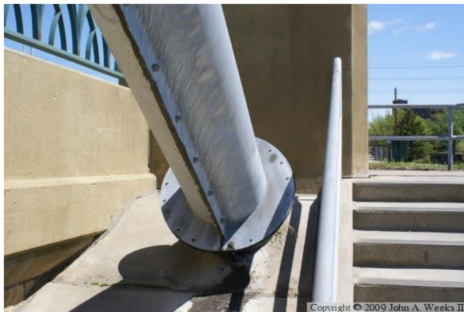
Figure 45: Example of Arch-Foundation Connection
