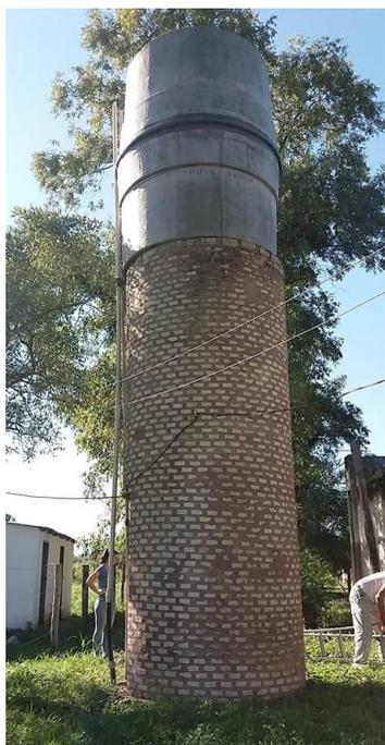
appeared to be relatively clear inside the tank, although there was some algae growth that seemed to be near the opening in the lid shown by the second photo. The water tank is supported by a hollow cylinder made of brick and mortar,
