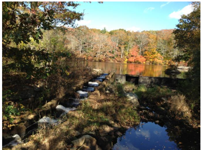
Figure 1: Russells Mills Dam
