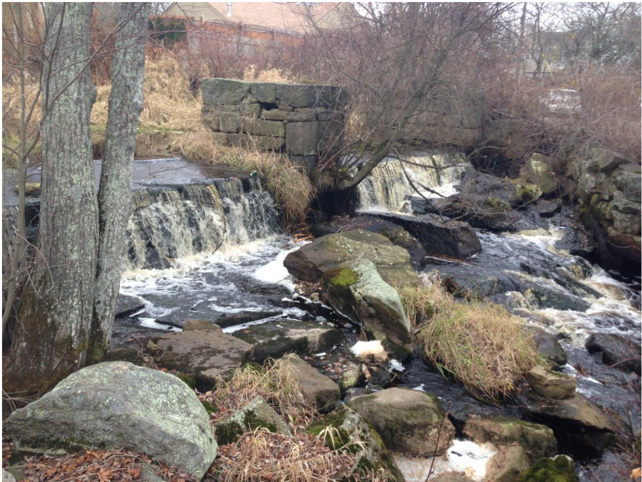
Figure 13: Smith Mills Dam
