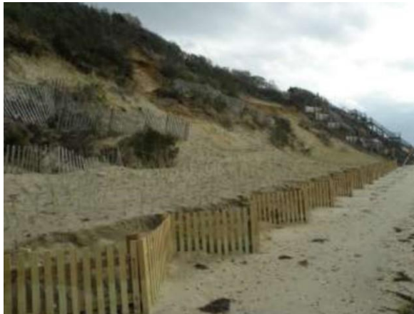
Figure 6: Sand Dune with Beach Grass and Fencing on Nantucket (Hunt et al. 2014)
