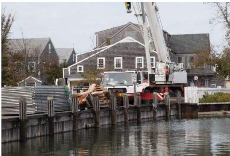
Figure 16: Easy Street Bulkhead Repairs (Pykosz, 2016)
