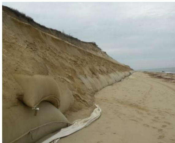
Figure 5: Geotubes in Sconset, Nantucket (Hunt et al. 2014)
