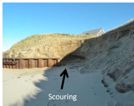
Figure 7: Scouring at End of Seawall on Nantucket (Hunt et al., 2014)
