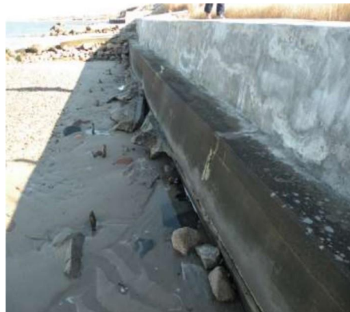
Figure 2: A Seawall on Quaise Road, Nantucket (Hunt, Sample, & Sullivan. 2014)
