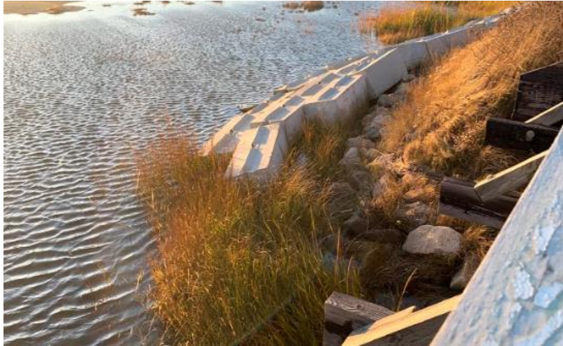
Figure 23: Jersey Barrier Below Millie's Bridge (Keable, 2019)
