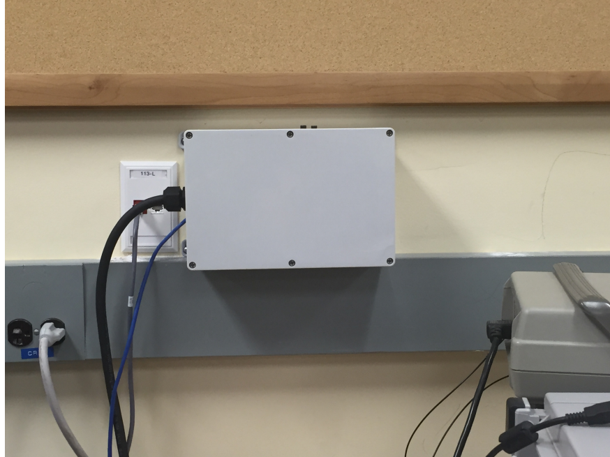
Figure 84: Installed Box in AK113
