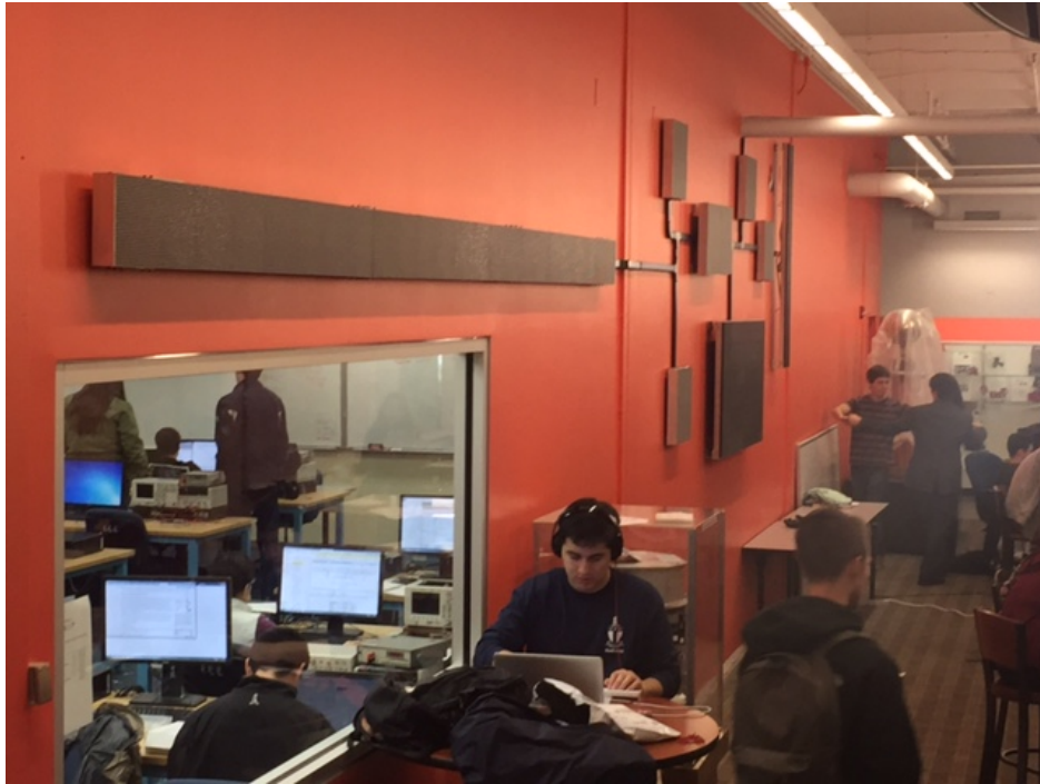
Figure 79: Power Panel in Pumpkin Lounge
