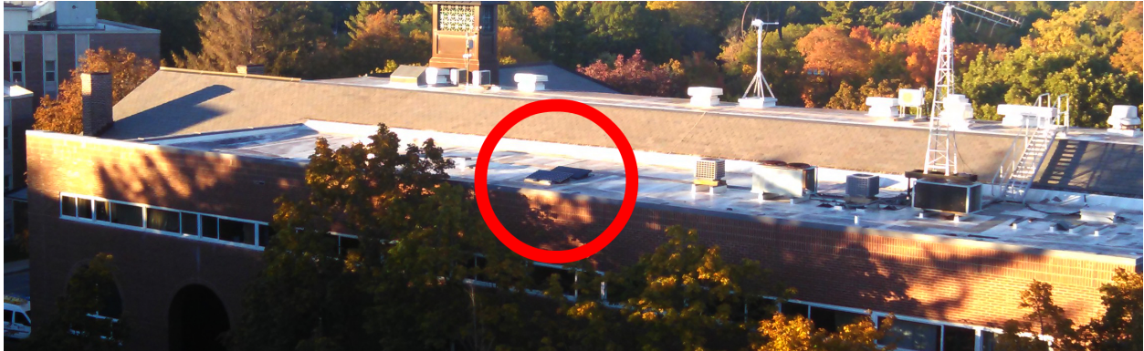
Figure 2: Location of Solar Panels of Roof of AK
