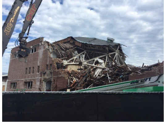
Figure 3 Alumni Gym During Demolition, August 2016
