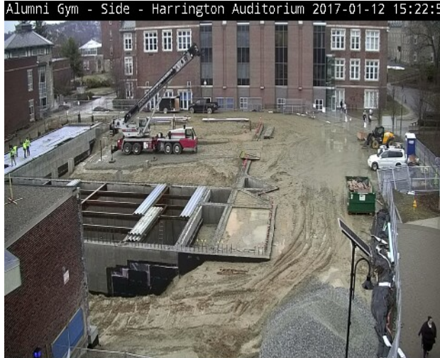
Figure 12 Actual Project Progress as Taken by Surveillance Camera
