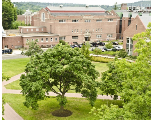
Figure 2 Alumni Gym Before Demolition
