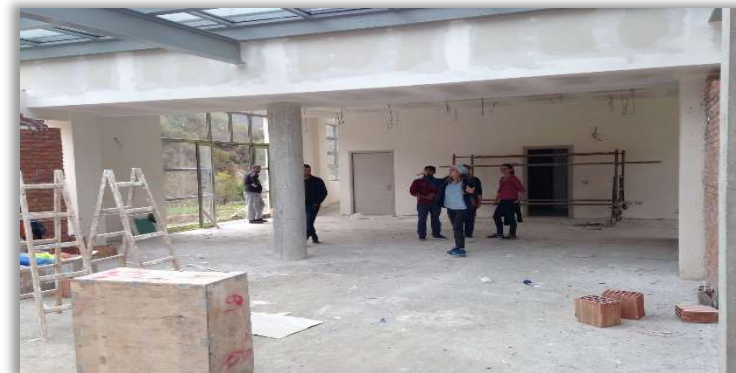
Figure 11: Building 1 at ARG Site
