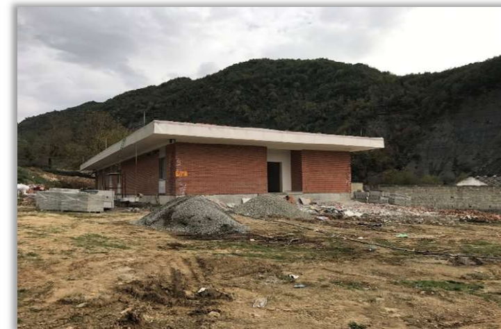
Figure 12: Building 4 at ARG Site
