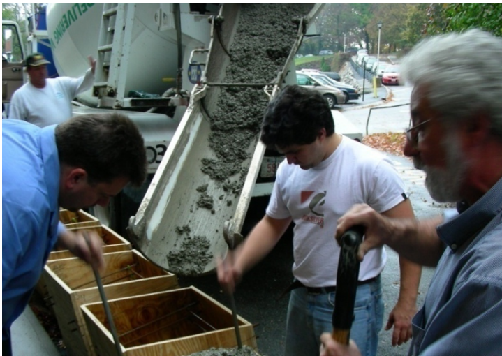
Figure 12 Concrete Pouring into Wood Molds
