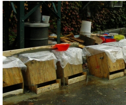
Figure 11 Concrete Block Construction Process.
