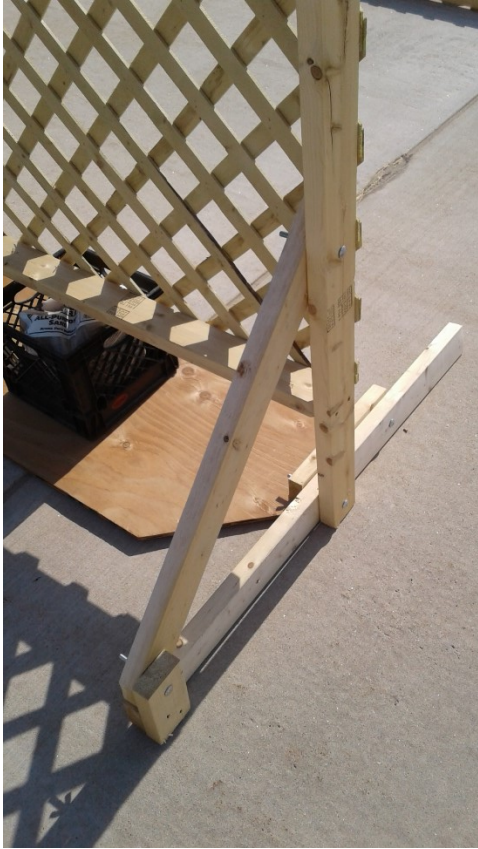
Figure 19: Attaching the gusset
