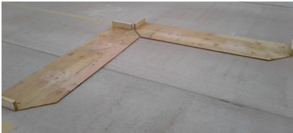
Figure 21: Base plate corner alignment
