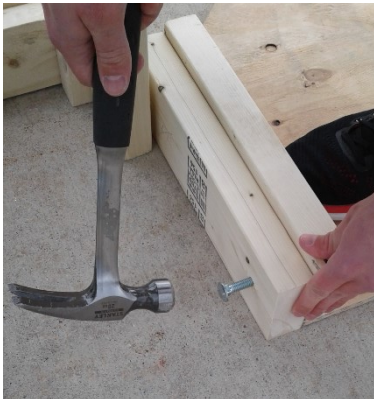
Figure 17: Driving bolts
