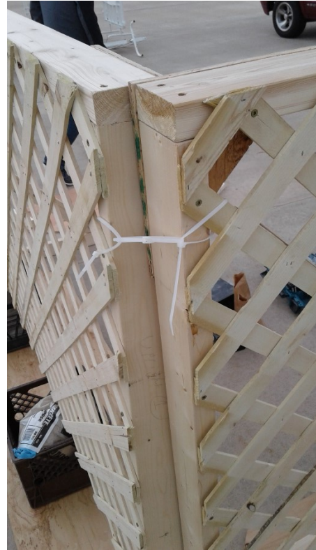
Figure 24: Securing corners with zip ties
