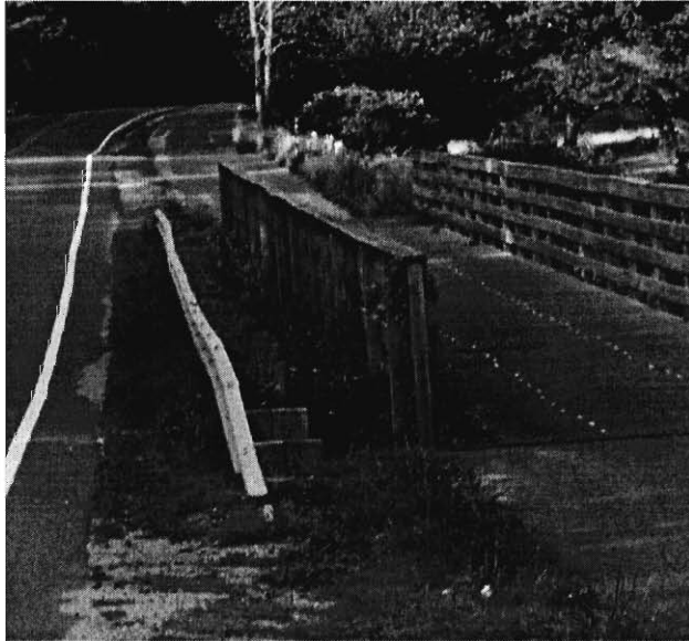
Figure 7: Bridge on Edgartown - W. Tisbury Road
