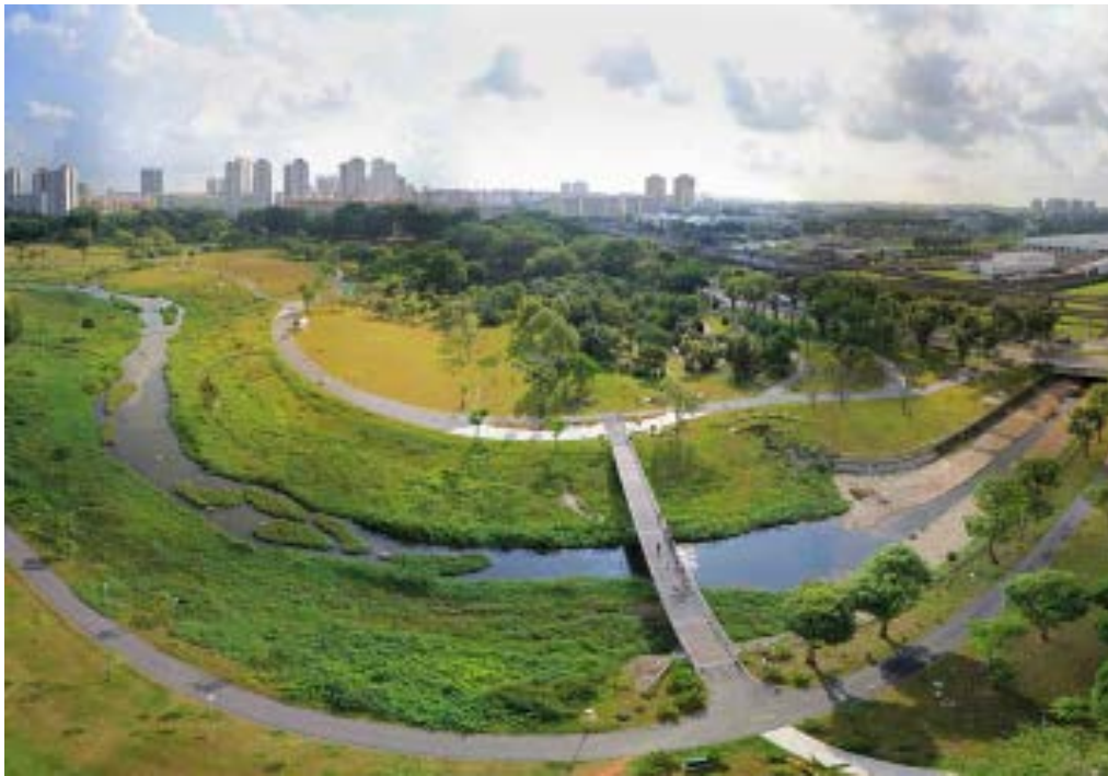
Figure 11: The renovated Bishan Park, Singapore (CH2M Hill, 2012).
