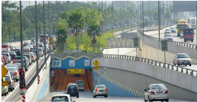
Figure 7: Picture of the SMART traffic tunnel (Gamuda, 2012).
