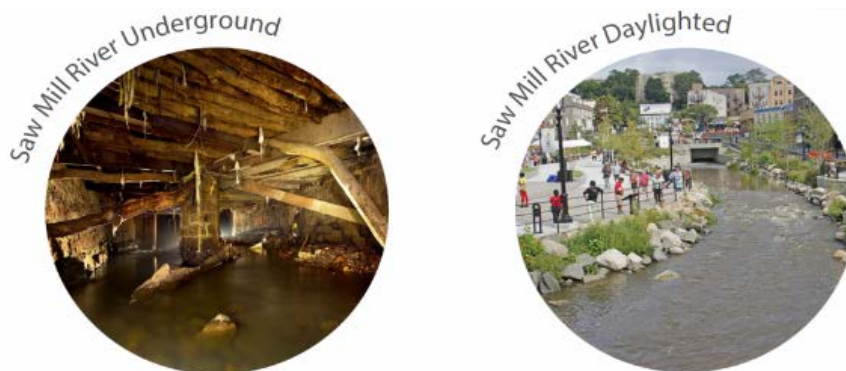
Figure 10: The buried Saw Mill River and the recently daylighted portion (Kramer, 2014).
