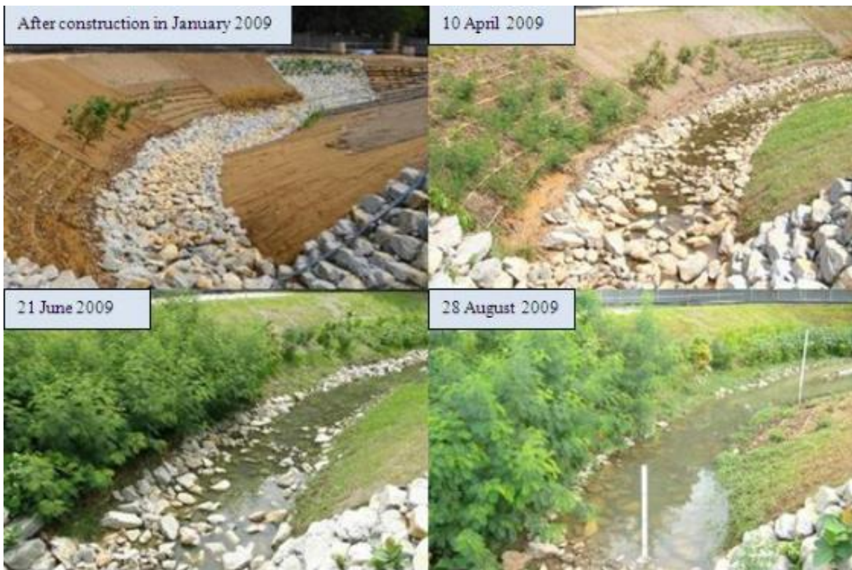
Figure 12: The 60 meter test bed in Bishan Park, Singapore (Public Utilities Board of Singapore, 2010).
