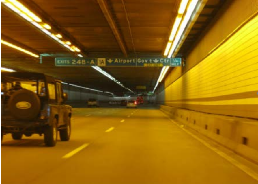
Figure 4: Inside the Ted Williams Tunnel, Boston, Massachusetts (Adderly, 2013).
