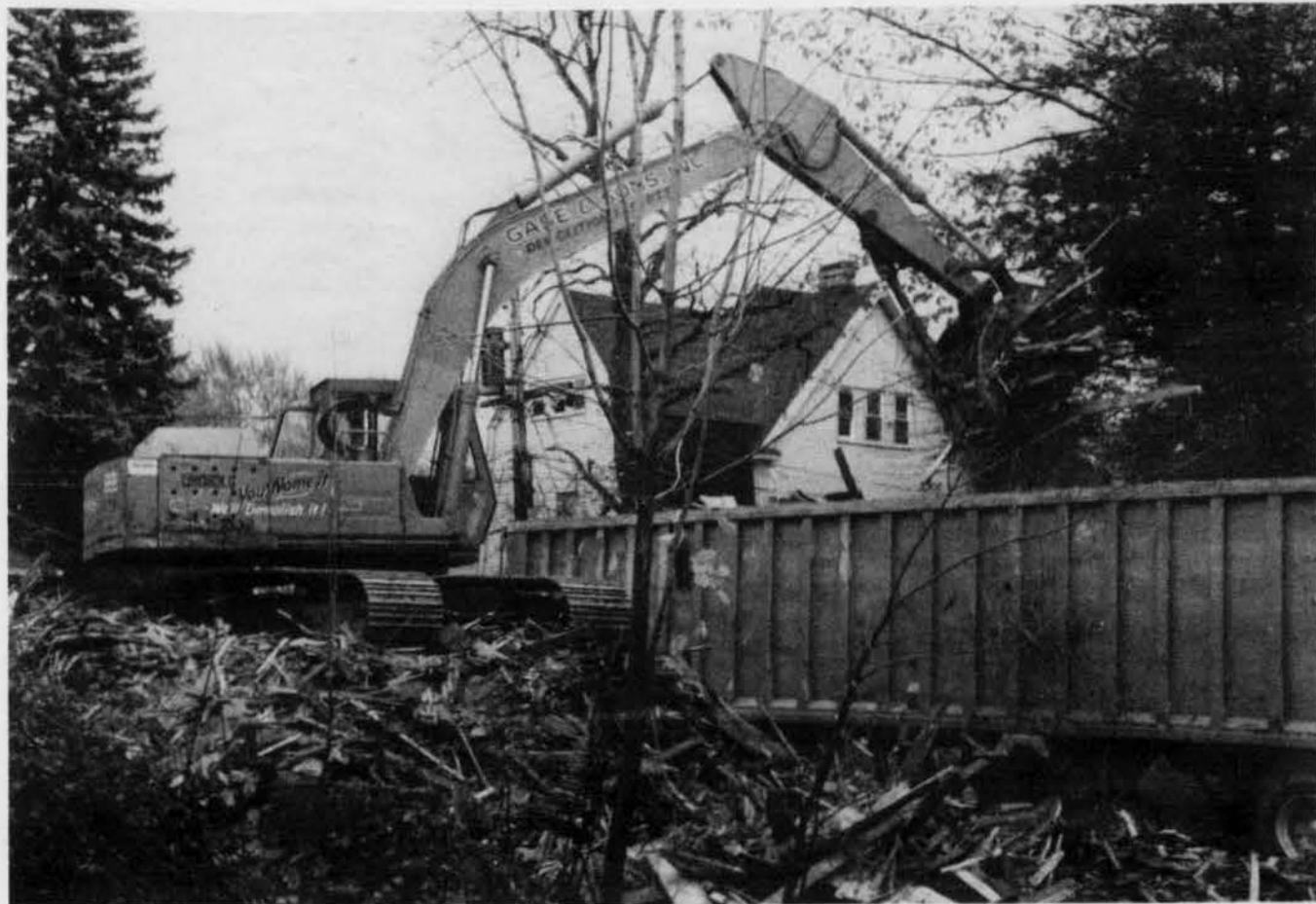
Demolition of KAP house
