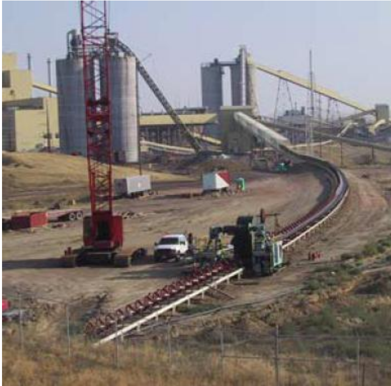
Figure 3. Curved Conveyor (Alspaugh M. , 2004)
